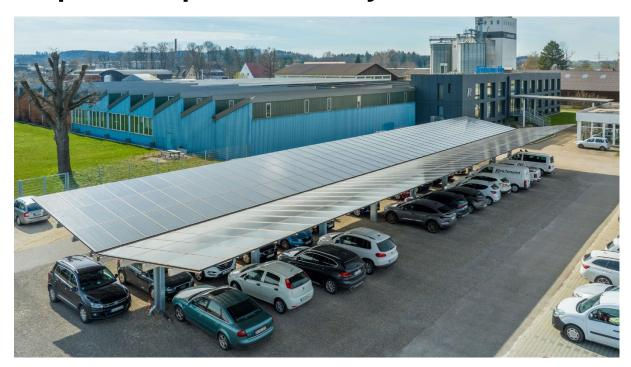
Reichmann & Sohn GmbH has made a sustainable investment in the car park of its company premises. The newly built carport with a photovoltaic system integrated into the roof covers more than half of the company's annual energy consumption. An extension is already being planned.
